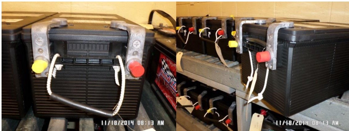
SIDE POST BATTERY PN# 908DFT716 DEKA or Approved Equal
